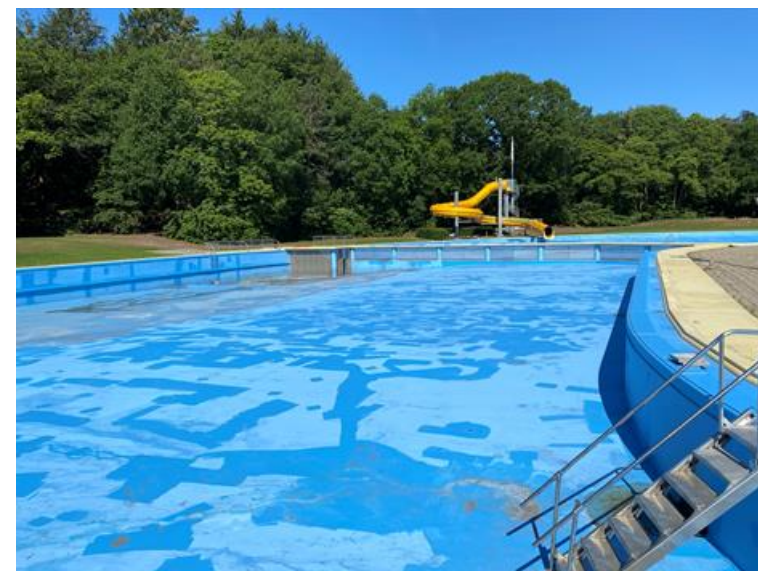
Figuur 16: Recent herstelde coating in bassin
